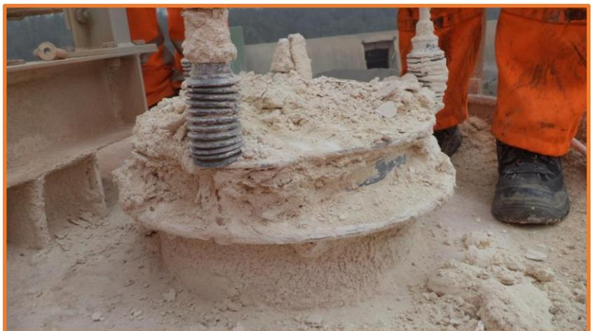
up. Unfortunately many maintenance engineers just don't realise the potential dangers that lurk beneath. They often think that simply cleaning off the material on and around the PRV is good enough. They don't realise that if the PRV doesn't lift next time an 'event' occurs, the over-pressure could easily rupture the silo or eject the filter housing from the top. On an ATEX-rated silo the over-pressure could
