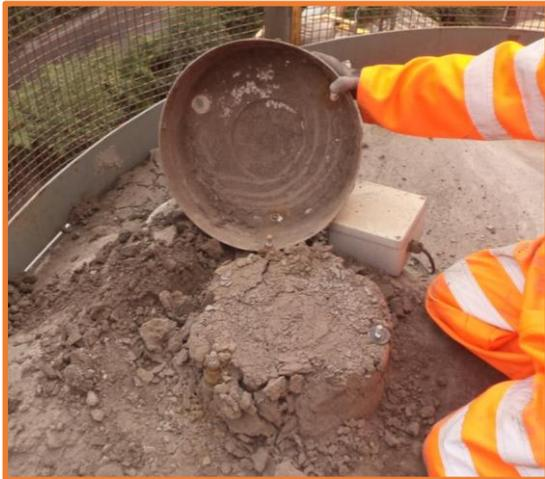
Silo protection systems are designed to prevent the damaging and potentially dangerous consequences of silo over-filling or over-pressurisation when powdered material is being transferred pneumatically from road tankers to silos. Unfortunately, perched out on the top of silos, such protection systems are all too often ‘out of sight, out of mind’ – until a major problem occurs!
