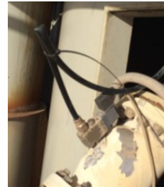
Above: this airline has been kinked to bypass the valve
