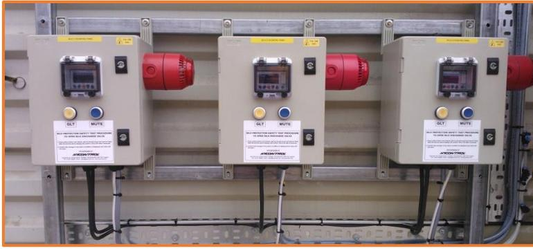
Diamond Point vibrating probe on a 1m-long cable providing the HLA, a FLEX501-D pressure sensor and a bespoke alarm panel with GLT capabilities and auto shut off.
