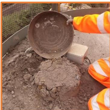
Pressure relief valves that, while dusted off on top, have not been pressure-tested or even had the lid removed to clean the valve. Frequently these valves have become blocked with product blown out of the silo (typically due to blockages in the filter or uncontrolled filling procedures). In one recent case, Hycontrol engineers found large deposits of moss growing underneath the lid of a PRV that had just been 'serviced' the previous week.
